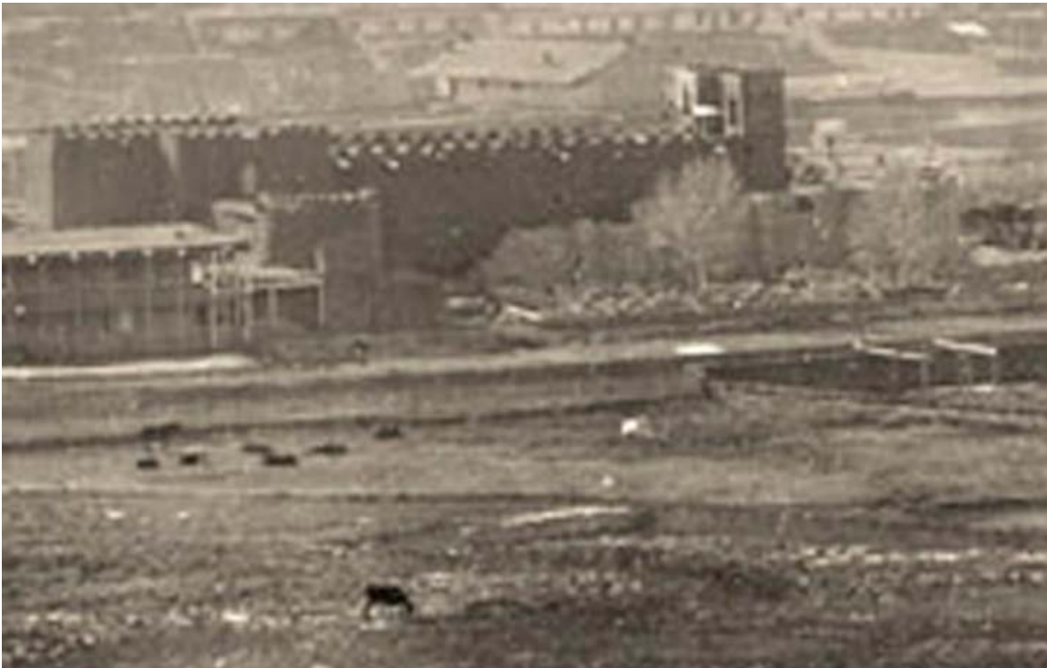
Beginning of construction, 1873 Photographer – Timothy O'Sullivan
