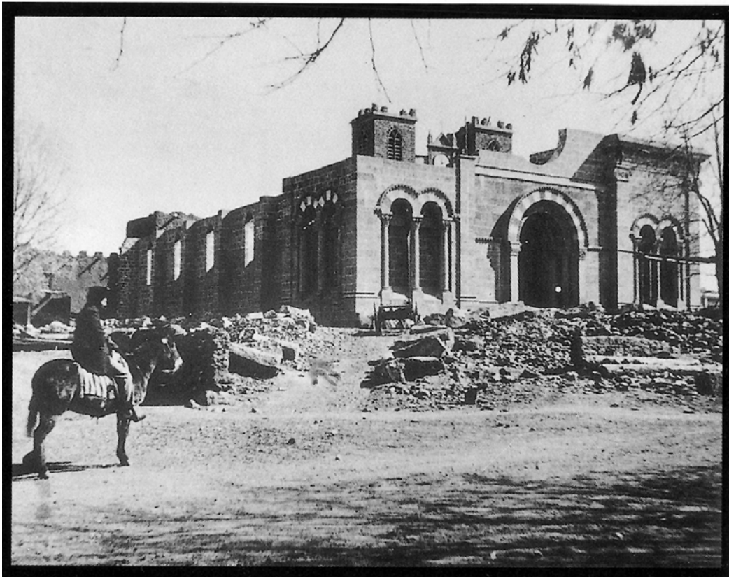
Construction continues, late 1870s
